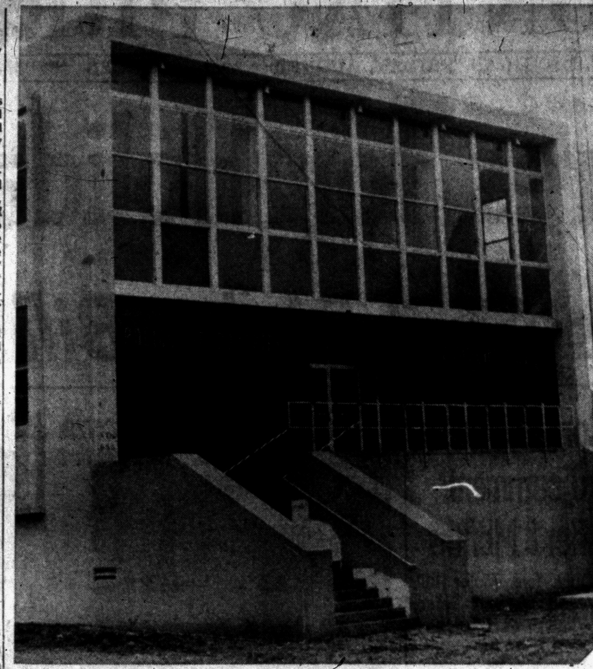
NEARING COMPLETION — This is the Pike street and main entrance of the city's new Public Safety Building. Leo J. Heenan, architect for the $375,000 structure, yesterday said the contracting work would be completed within a week. Acting City Manager Lewis M. Wrenn said he expected partial occupancy by the police department by Sept. 15. Besides the police, the building, next to the City Hall, will house two municipal courts and offices, and headquarters for the fire department. (See other pictures on Page 2L)
