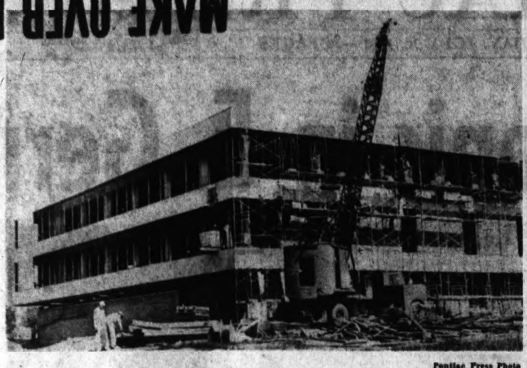
MEETING THE TIMETABLE—This is the future $1.5-million Krueger Library of Michigan State University. Scheduled for completion this fall, the building will house 300,000 volumes—and can be tripled in size by additional wings. Workmen are currently finishing out-side brick work, installing elevators and working on the electrical system of the building. On the highest ground of the campus, the library will be MSU's dominant landmark.
