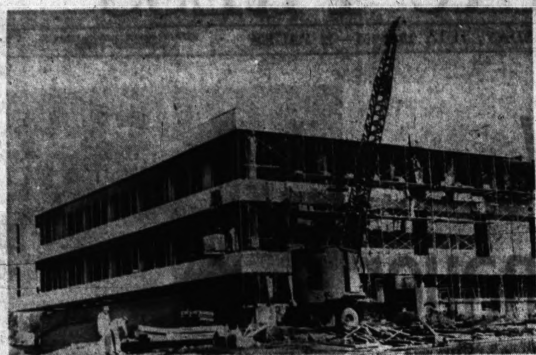
MEETING THE TIMETABLE—This is the future $1.5-million Kresge Library of Michigan State University. Scheduled for completion this fall, the building will house 300,000 volumes—and can be tripled in size by additional wings. Workers are currently finishing out side brick work, installing elevators and working on the electrical system of the building. On the highest ground of the campus, the library will be MSU's dominant landmark.
