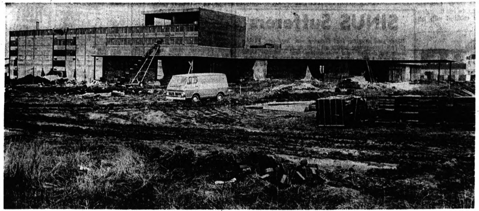
ON SCHEDULE — Work on the Sheraton Motor Inn on Woodward across from St. Joseph's Mercy Hospital in Pontiac is right on schedule. The inn is expected to open by July 4, according to Charles Langs, developer. The $2.5-million facility will contain 158 rental units and dining room accommodations.
