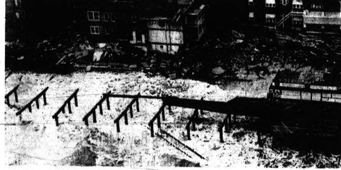
BOARDWALK RIPPED UP — Vacationers who have strolled along Atlantic City's famed boardwalk would have trouble recognizing it today. Planks are shown here strewn against oceanfront homes after being ripped from their pilings by monstrous tides that lashed the Eastern Seaboard earlier this week. At least 35 persons have been killed in the storm and many others are missing.
