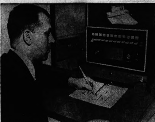
NEW TECHNIQUE — Using a special electric pen, a man writes on a tablet during a demonstration of "blackboard-by-wire." The technique utilizes ordinary telephone lines for transmission to television receivers. A voice is carried by a separate telephone line.
