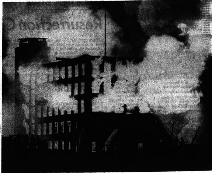
NINE-ALARM FIRE —Flames shoot from a paper box manufacturing firm's plant in Philadelphia last night.
