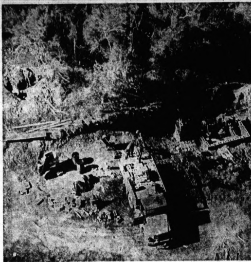
FORTIFICATION BUILD-UP — Marines on the Guantanamo Naval Base construct new fortifications. This air view shows Marines unloading cinder block from a truck
