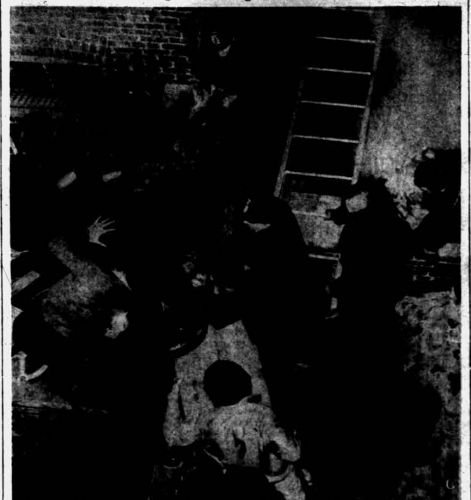
TEAMWORK—Firemen in Baltimore hurry as they remove one of their men from the wreckage of a clothing store fire. Six firemen are feared dead after they were trapped when the roof collapsed during the blaze.
