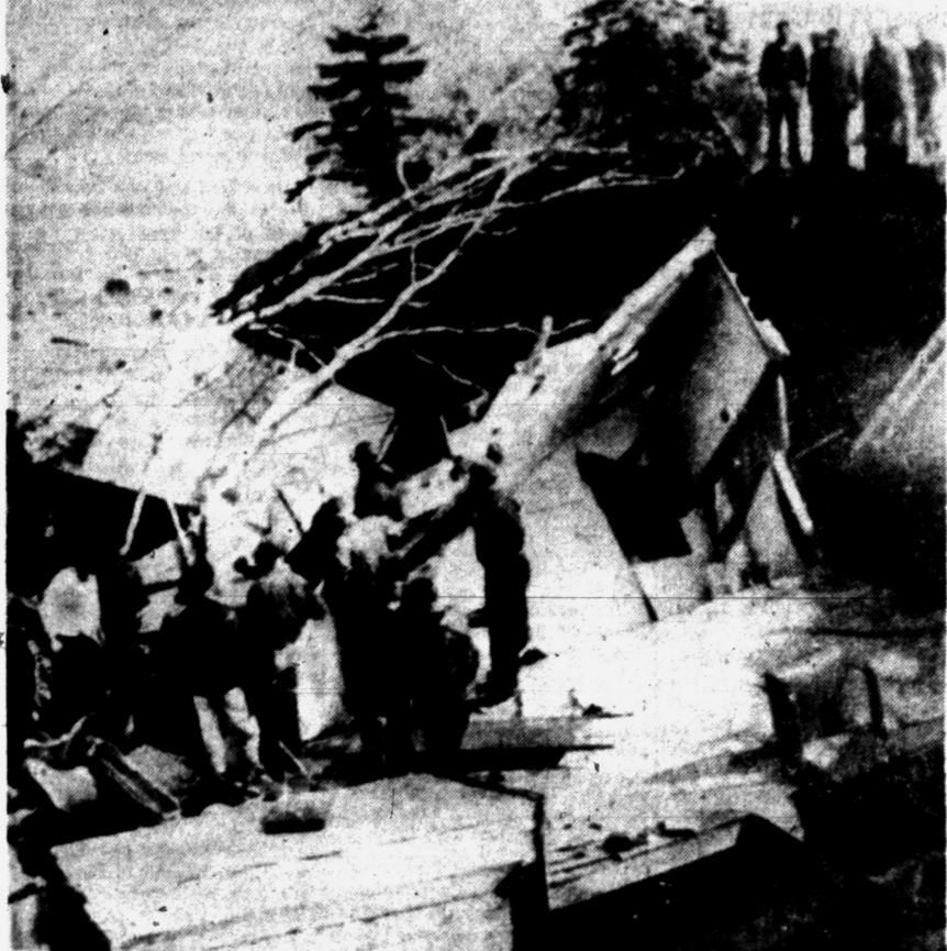
TOPPLES INTO WASHOUT — A windstorm accompanied by torrential rain toppled this house into a washout near Sault Ste. Marie, killing one person and injuring three others.
