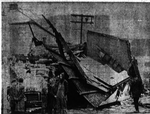
RELIC IN RUINS — The 217-year-old Rogers Daniels house of Newton Center, Mass., lies in a broken heap over a truck trailer that was carting it away from its original site to make way for a toll road extension into Boston. The
