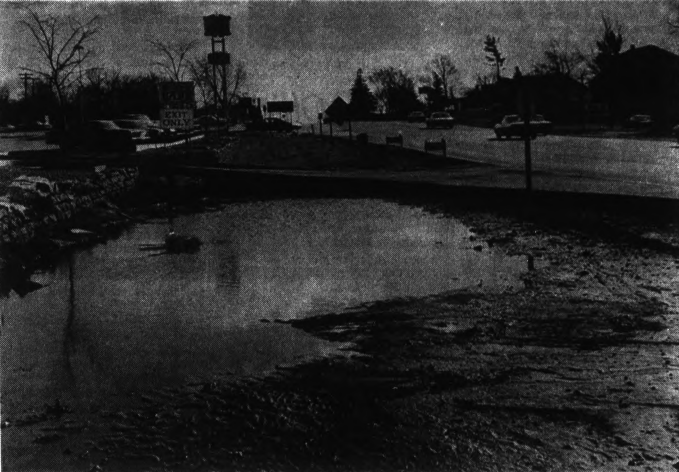
ROAD HIGHER, WATER REMAINS — State Highway Dept. workmen have raised Dixie 1 1/2 feet at this long-time trouble spot south of Walton. However the ponded water indicates the problem will be the same the next time water flows in the area. The drain under the highway, leading west, has been plugged for years and in times of heavy rain or melting snow the road floods and hinders passing traffic as well as flooding adjacent property.
