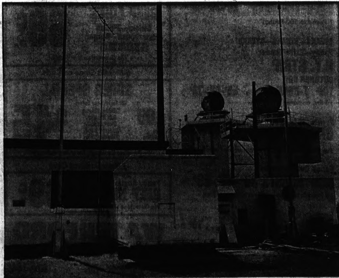
Fire Control Area Of The Shelby Township Nike Base
