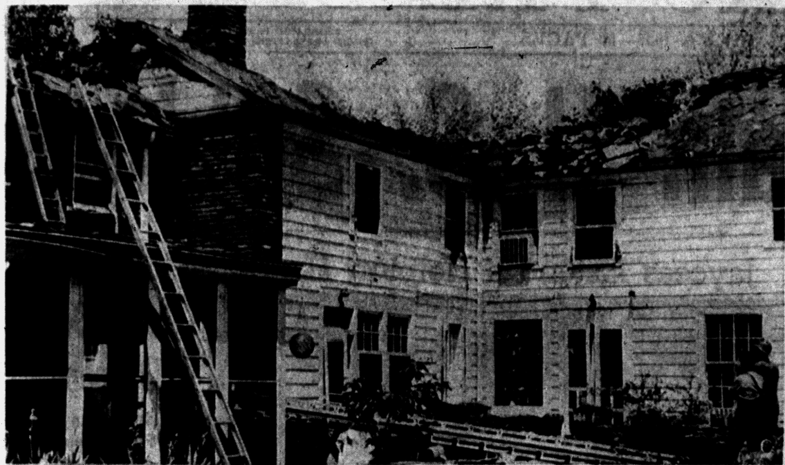
$50,000 FIRE IN BIRMINGHAM —Damages caused by a fire Saturday morning at the home of a prominent Birmingham psychiatrist and author, Dr. J. Clark Moloney, 414 Arlington Rd., were estimated today at $50,000. The blaze started in the incinerator
