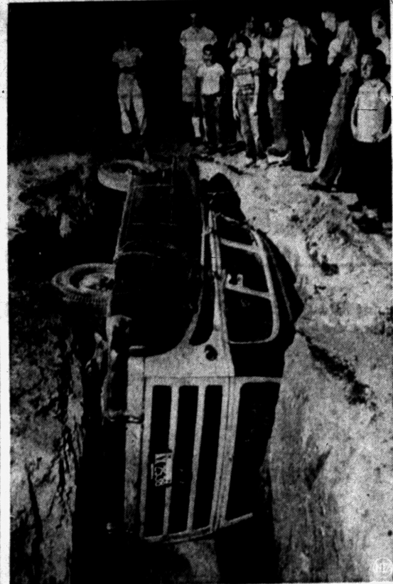
SQUEEZE PLAY — Sixteen-year-old John Eldred didn't mean to "park" his car in this awkward position in Indianapolis, Ind. He accidentally bypassed a "road closed" sign, and the car ended up wedged sideways in the ditch of a new storm sewer. Eldred squeezed unhurt from the car.
