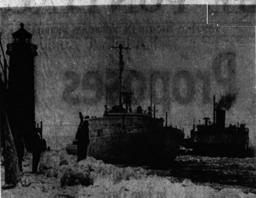
FREES ICEBOUND SHIP —The Mackinac, biggest icebreaker on Lake Michigan, opens ice-plugged Grand Haven Harbor to free the tanker Meteor today. The tanker was stuck since last Wednesday. The Mackinac escorted the tanker through a two-mile ice field to open water.
