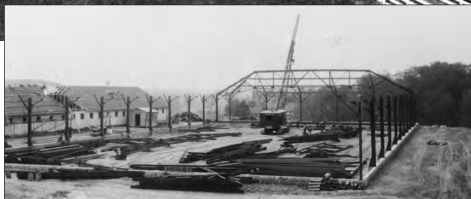
Top: Meadow Brook Farms equine complex, c. 1940: (left to right) horse stable and location of Frank’s construction office; Frances Dodge’s stable and Riding Ring, Matilda and Alfred Wilson stable. Bottom: Riding Ring under construction, c. 1935.
