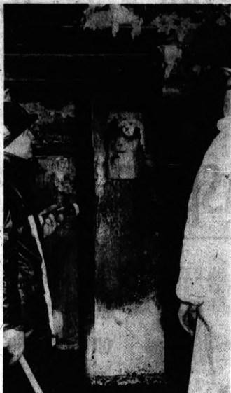
PROBE DAMAGE —Bloomfield Township fire fighters investigate damage inflicted in a $4,900 home fire late yesterday afternoon at the home of W. J. Simons, 784 Woodlake. No one was injured.
