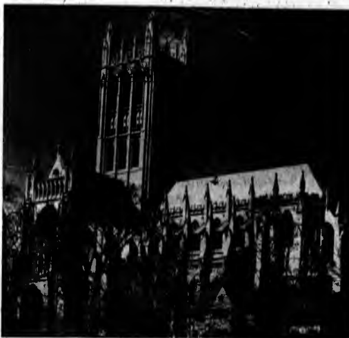
WASHINGTON CATHEDRAL — The view from the southeast shows the recently completed Gloria in Excelsis Tower of Washington Cathedral, Washington, D. C.
