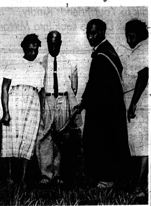
BREAKS GROUND — Dr. J. Allen Parker turned the first shovel of earth in groundbreaking ceremonies for Newman AME Church this week. Also participating were (from left) Mrs. Ralph St., general chairman. The new church will be located at Brush and Bagley Streets.
