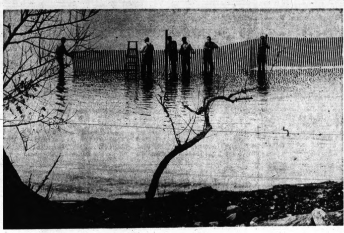
SNOW JOB? — That's a snow fence worker putting up in Orchard Lake. In past winters, Oakland County Road Commission officials were unable to solve the problem of snow drifting over the ice, across a dangerous curve in Orchard Lake Road. The road at this point is between Pine Lake and Orchard Lake. It is steeply banked on both sides, with no place for a snow fence. A crew put up this 300-foot-long snow fence yesterday in the lake about 25 feet from shore. County road officials think they have solved the problem.
