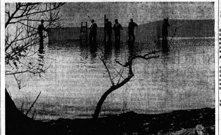
SNOW JOB? — That's a snow fence workers are putting up in Orchard Lake. In past winters, Oakland County Road Commission officials were unable to solve the problem of snow drifting over the ice, across a dangerous curve in Orchard Lake Road. The road at this point is between Pine Lake and Orchard Lake. It is steeply banked on both sides, with no place for a snow fence. A crew put up this 300-foot-long snow fence yesterday in the lake about 25 feet from shore. County road officials think they have solved the problem.
