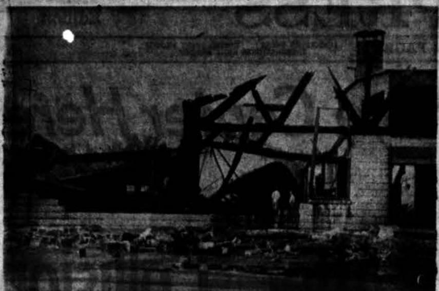
DESTROYED BY FIRE —All that remains of the production section of the Oakland Foundry and Machine Company on Woodward Street in Rochester is shown above. The building was destroyed by fire of unknown cause during the night. Damage estimates range between $75,000 and $100,000. Two other buildings of the plant were untouched.
