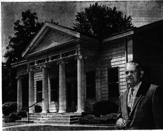
LOOKS OVER BUILDING - Checking the roof and siding of the First Church of Christ, Scientist, 164 W. Lawrence is Rufus Campbell of 4128 Quillen, Waterford Township. Mr.
