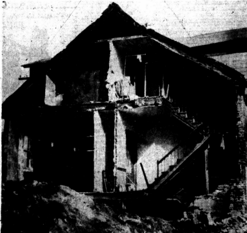
DOLL-HOUSE STYLE — This home of Mrs. Sarah Suddeth of Wellsburg, W. Va., was reduced to three walls recently when Floyd Adams razed a house which shared the south wall of the Suddeth home. Mrs. Suddeth has filed a $10,000 damage suit, and the family is living in half of the house.
