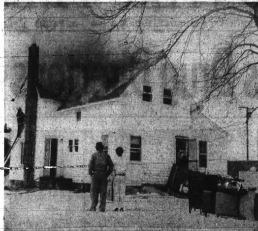
SECOND STORY GONE — A fire of undetermined origin demolished the second story of this white frame house in Brandon Township yesterday. Damage was estimated at $4,000 - $6,000. But through the efforts of fast-acting neighbors and the Ortonville Jaycees, most of the contents were salvaged. Oxford fire fighters assisted by Brandon and Lake Orion fire departments. The house, owned by Carl W. Bower, is at 5401 Sherwood Road.
