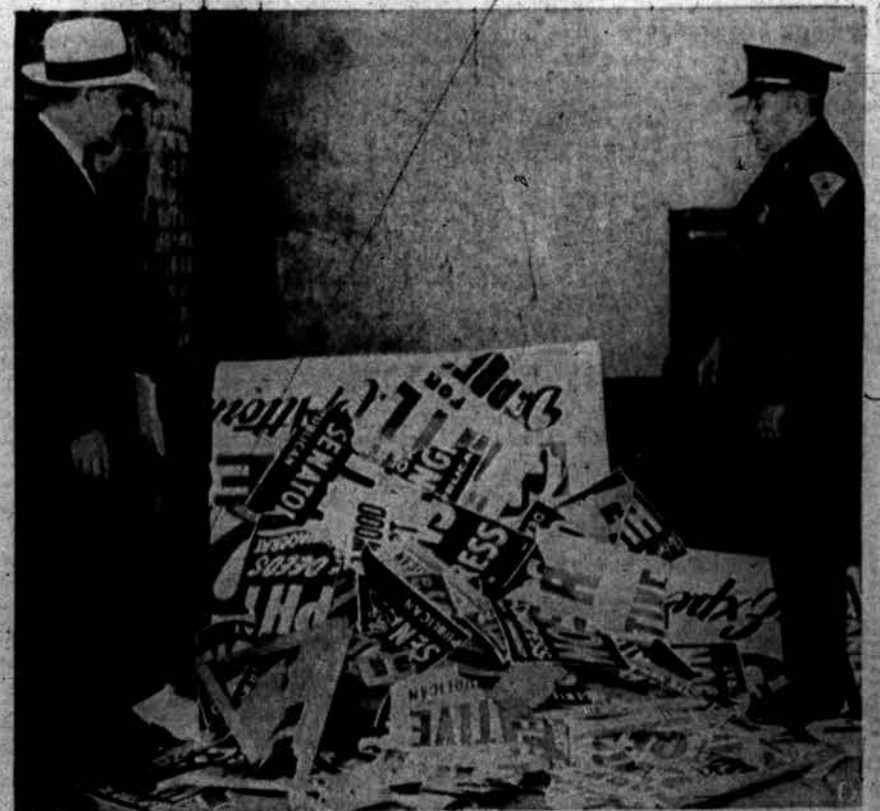
'IT AIN'T LEGAL, MISTER' — Pontiac Police Chief Herbert W. Straley and uniform Captain William Crisp eye a pile of confiscated political signs which blossomed on utility poles and public property in the city in violation of a city ordinance. According to Straley, this is the second such pile of signs torn down by police since the current campaign started. There's a $10 fine or 20 days in jail waiting for anybody caught putting up an illegal sign, the Chief says.
