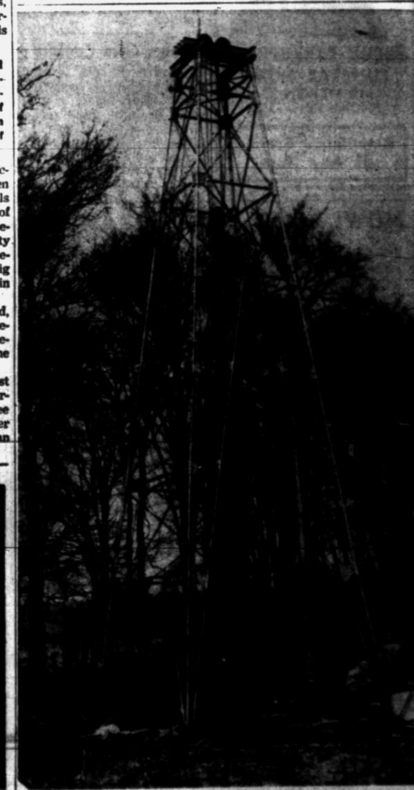
NEW CITY WATER WELL—A crew is shown drilling the first of three new water wells near Silver Lake. The wells are expected to up Pontiac's potential water supply about 25 per cent and produce an estimated 2,700,000 gallons a day. The wells will cost about $80,000. City officials hope the wells will be in operation before summer's peak demand.
