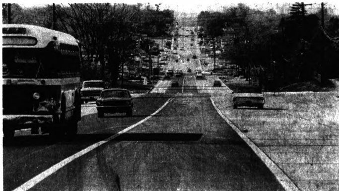
DETROIT ENDS — After being closed to all but local traffic for four months while being improved, Elizabeth Lake Road between Josephine and M59 in Waterford Township is now open to all through traffic. The modernization of the one-mile stretch includes the widening of the roadway from two
