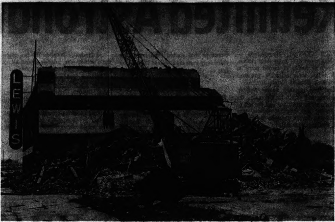
DOWNTOWN BUILDING RAZED—Demolition of the Lewis Furniture building began yesterday and is scheduled to be completed this week. The building, last in the city's central business district to be demolished for the city's urban renewal
