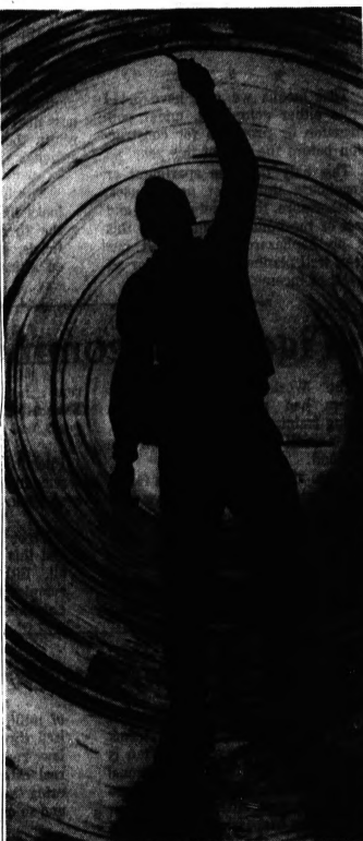
IT STACKS UP — Charles G. Diehm of New Castle, Del., inspects the interior of a seven-foot-diameter section of a fiber glass smokstack before it and two other sections, which will form a 285-foot stack, were loaded aboard barges for shipment to New Jersey.
