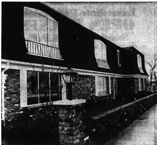
NOW RENTING — One and two bedroom apartments are available for rental at the Darling Court Apartments, 3440 Sashabaw, Waterford Township. Built by Leon Blachura of 3538 Pontiac Lake, Waterford Township; the building features 11 units. Each carpeted kitchen is furnished with complete laundry, cooking and dishwashing appliances.
