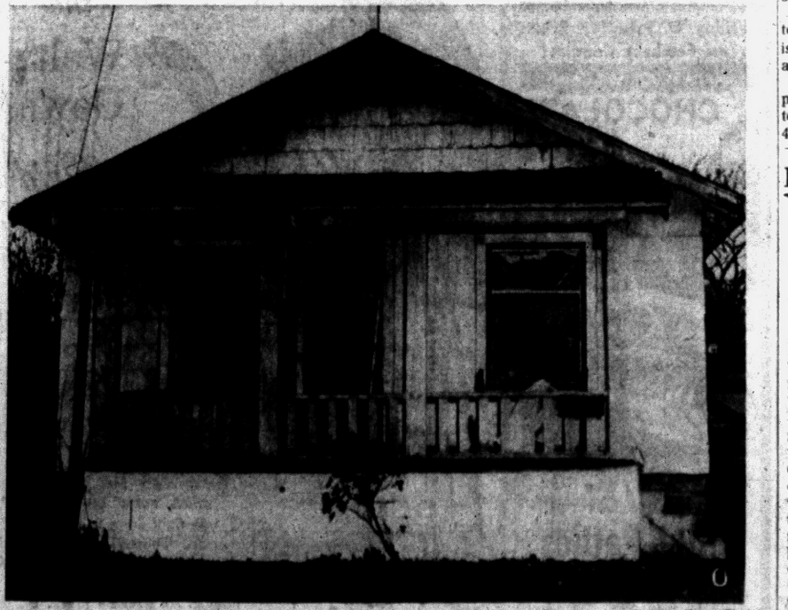
SHATTERED HOME —The frame home at 370 S. Edith that was ripped by an explosion this morning shows damage signs from the front. The broken window is in the bedroom of Mrs. Mae McGowan, who narrowly escaped injury by going into the living room seconds before the blast. The front door is partially blown off its hinges.
