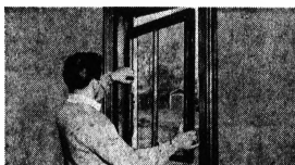
Old windows are easily replaced from inside. First, sash and cords are removed.
