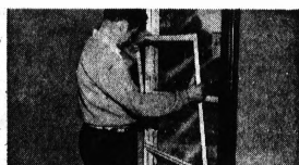
Aluminum Nu-Sash are snapped into place without disturbing plaster or woodwork.
