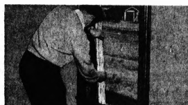
Insulated tracks are fitted into the sides of the window opening.
