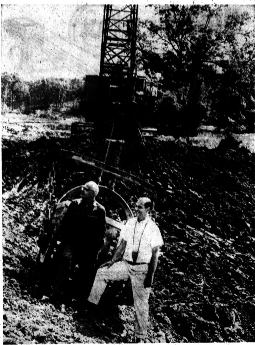
RIVER MAKER — One of Michigan's largest cranes is digging a 30-foot deep river at Silverbell Village, a year-round recreation area presently under construction on M24 near I-75 in Orion and Pontiac townships.
