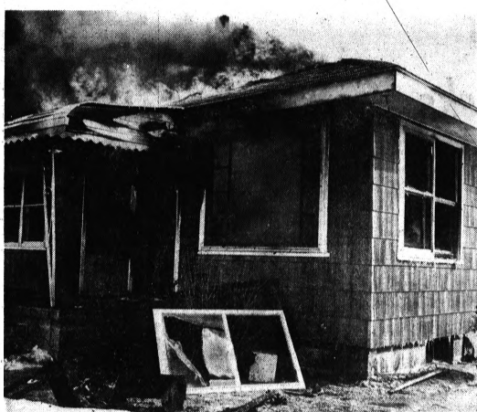
TOTAL LOSS — Fire of undetermined origin yesterday afternoon destroyed the frame ranch house of Edwin W. Kendall, 5011 Walden Road, Independence Township. Additional damage of from $3,000 to $3,500 was estimated on contents. Independence Township fire fighters were aided by firemen from Waterford Township battling the blaze in near-zero temperatures.
