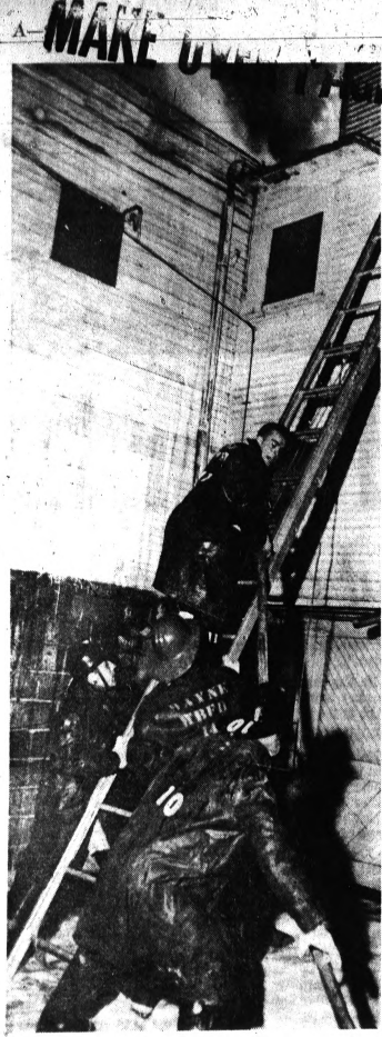
Teamwork at Keego Fire
