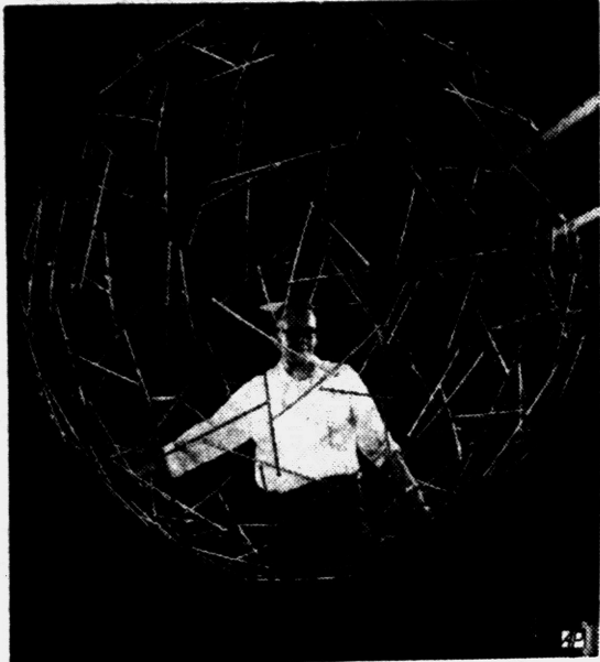
STRONG BALL — Student stands within "discontinuous sphere" at Carbondale, Ill. school. None of 270 parts touches another. Design can support great loads.
