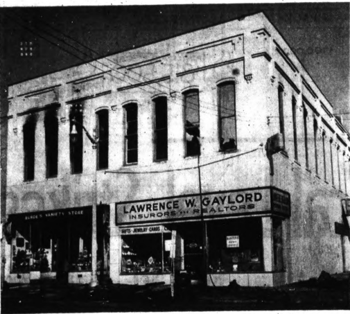
AFTERMATH OF FIRE — The Masonic Temple on the second floor of this two-story brick structure in the heart of Lake Orion is open to the sky today after being gutted by fire early yesterday morning. The two busi-
