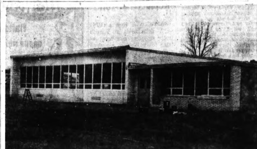
MISSION BUILDING —St. Daniel's, a mission of Our Lady of the Lakes Church, Waterford Township, under construction at Miller and Holcomb, Clarkston, is slated for completion in January. The $929,000 building will
