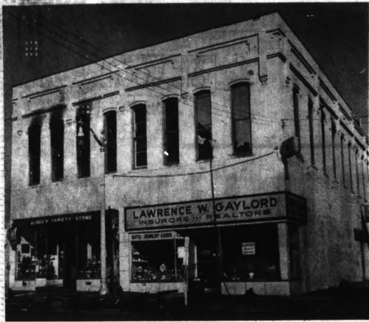
AFTERMATH OF FIRE — The Masonic Temple on the second floor of this two-story brick structure in the heart of Lake Orion is open to the sky today after being gutted by fire early yesterday morning. The two businesses on the floor below were damaged extensively by water pouring into the building. Nine area fire departments brought the blaze under control in about four hours.
