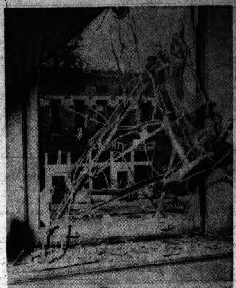
RUINED WINDOW — A twisted, broken stained glass win- dow in the 16th Avenue Baptist Church illustrates the damage done by a bomb which blasted the building in Birmingham, Ala., yesterday. Four small girls were killed, and several were in- jured.
