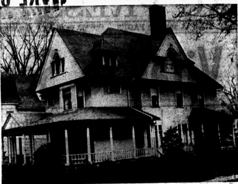
FOR CHILDREN — The county is turning this large frame home at 52 Franklin Blvd. into living quarters for 15-20 homeless children who otherwise would have to stay at the county children's home. When reconducted, the new facility will help relieve crowded conditions at the institution, a fact that will be emphasized when Oakland County Children's Home opens its doors for open house from 1 to 5 p. m. Sunday.
