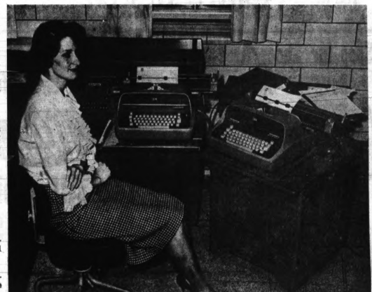
ELECTRICAL TYPISTS — New installations of specialized office equipment are adding to the efficiency of paper work in the business office at Pontiac State Hospital. The units save many hours of work, even if they are replacing the need for good looking stenographers. One of the good "old fashioned" type of typists, Mrs. Patricia De Longchamps of 6914 Tappan Court, Clark-
