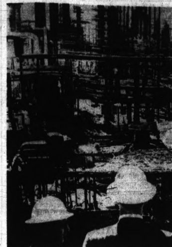
VIEW BLAST SITE —Plant officials look over the site of the flash explosion in a fractionating unit of the Phillips Petroleum Co. gas plant at Borger, Tex., Wednesday. Nine employees of the Bowman-Chase Construction Co. were killed and one injured.
