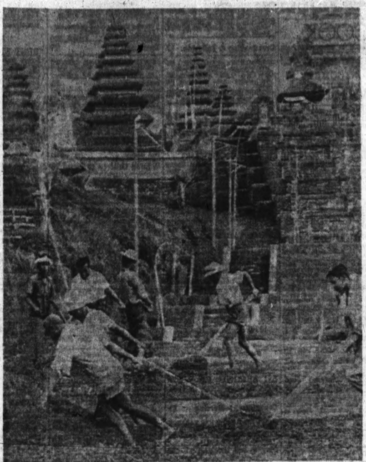
CLEAR BALI —Workers clear away 16-inch deep piles of ash and debris from background are pagoda-like temples, four recently erupted Agung volcano in Bali. In miles from the volcano.
