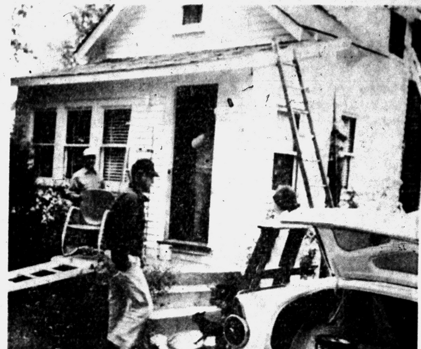
JAYCEES PAINT — Fourteen members of the Waterford Township Junior Chamber of Commerce welded paint brushes last Saturday, completely covering the home of Mrs. Mary Goodwin.
