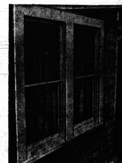
AFTER: Nu-Sash, installed here, had economically updated home, made tight against weather, never needs paint.
