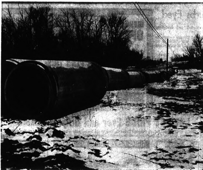
AWAITING CONNECTION — These hefty concrete cylinders, littering an open field north of Avon Road between Livernois and Rochester roads in Avon Township, will become part of the massive $28.2-million Clinton-Oakland Interceptor Sewer,
