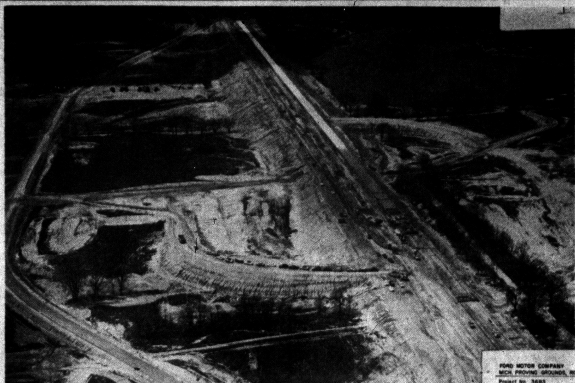
AERIAL VIEWS — Pictured above is network of roads looking west at one million yards of fill upon which will be placed a concrete, high-speed track and straightaway. Also visible is a section of basic durability road, and straightaway and high-speed access ramps.
