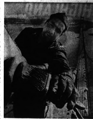
NERVES OF STEEL — Ray Santana of San Francisco is one of 40 elite painters who scramble daily 746 feet above the waters of San Francisco Bay to protect the famous Golden Gate Bridge. The crew continuously paints its 10 million square feet of deck, towers, supports and cables.
