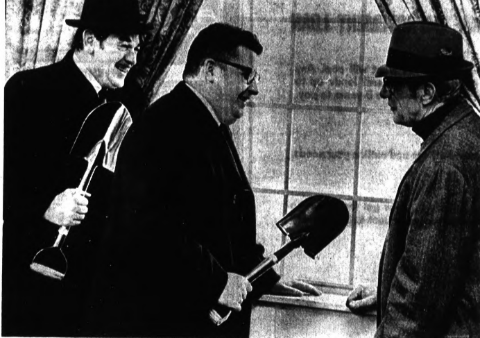
GROUND-BREAKING—Walled Lake City Manager Royce L. Downey (left), Mayor Wendel G. Kellogg Jr. (center) and R. J. Alexander, director of the Oakland County Department
