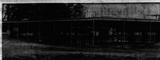
CONSTRUCTION CONTINUES — Sept. 31 has been set as the completion date for Holley Computer Products, a subsidiary of Control Data Corp. The $1 million, 60,000-square foot plant is being built at the corner
