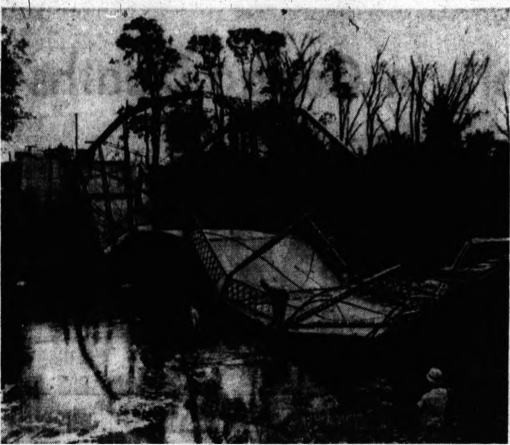
BRIDGE COLLAPSES — A skidding, runaway truck tore through the side of this bridge over the Cass River at the village of Tuscola in eastern Tuscola County a week ago, but the bridge refused to fall until yesterday. The 170-foot span collapsed as expected but caused no injuries, as it had been closed to traffic since the initial accident.
