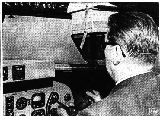
PHONY FOG — Simulated fog may help pilots improve their instrument procedures, particularly on landing approaches. Demonstrating is Paul Noxon of the Bendix Corporation's Navigation and Control Div., who is looking into a screen on which a fog pattern
