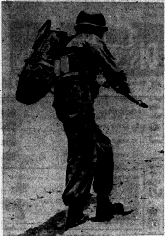
MOTORIZED GI — Sgt. Richard A. Quinn climbs hill wearing rocket-powered jump belt, designed to give infantrymen more mobility. The belt is a small unit strapped to his waist under his field pack. The jump belt is designed to assist in landing operations and jumping over obstructions which could not be covered in normal manner.
